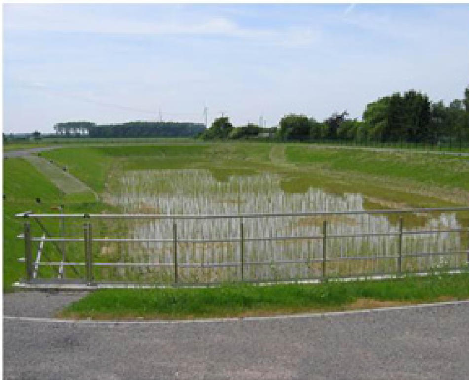
Figure 6: Retention basin (sedimentation) and retention soil filter for the disposal/treatment of storm water
